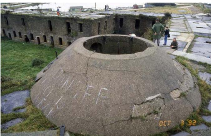
The concrete protection for the conning tower
